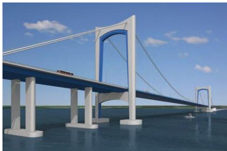
Figure 1 - Varvarovsky Bridge in 3D
